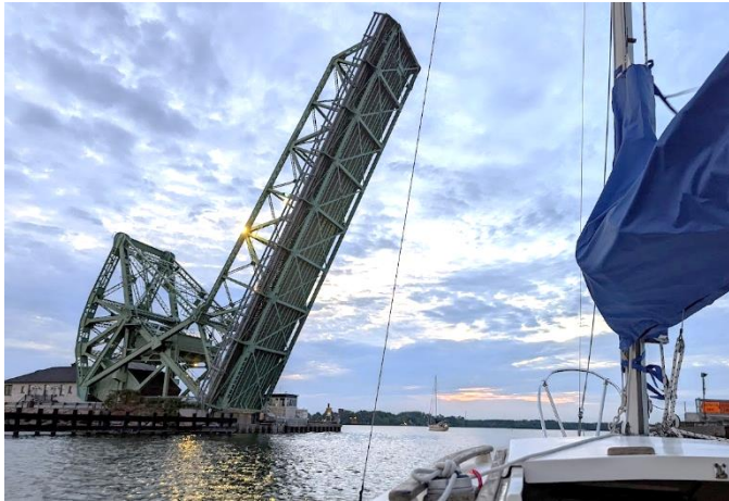
IMAGE: Bascule Lift Bridge, Lasalle Causeway Kingston ON
