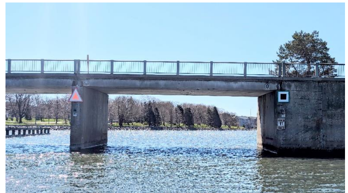
IMAGE: Concrete Span, East portion of Causeway.
